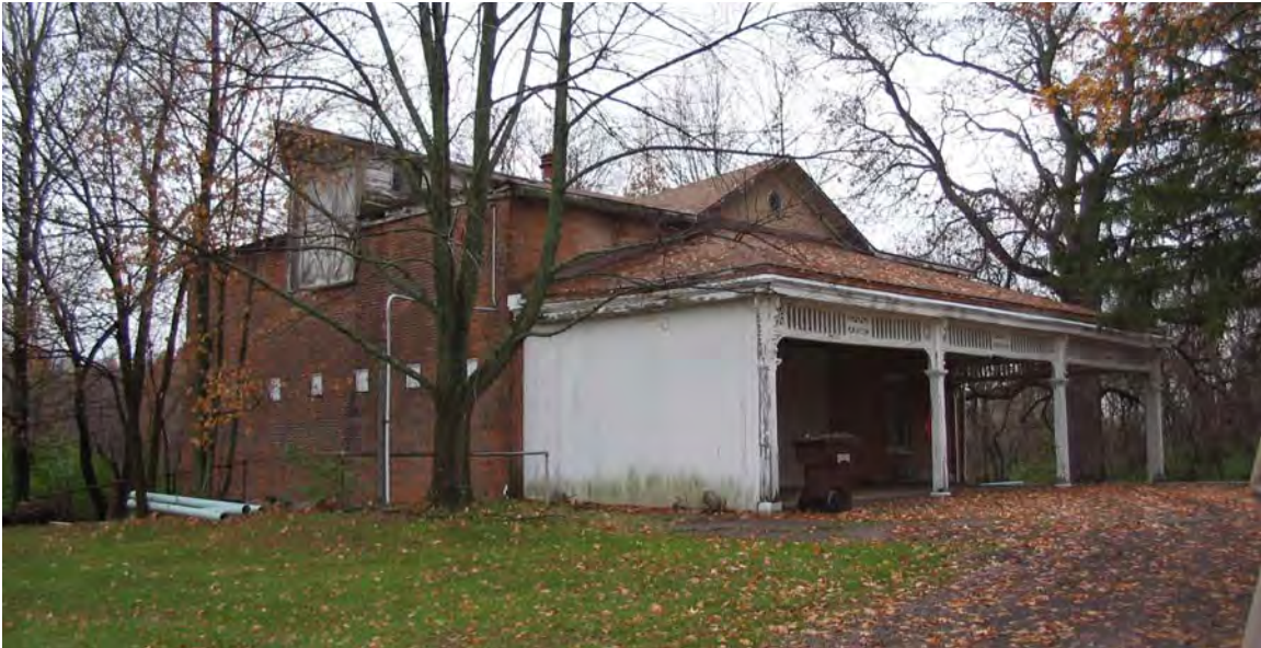
Photo 12. Carriage House, south and west elevations
