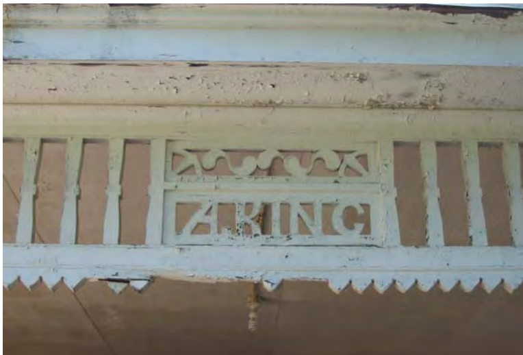
Photo 13. Carriage House, south porch detail
