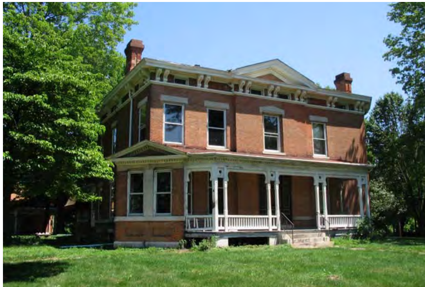
Photo 1. Front elevation, looking north
