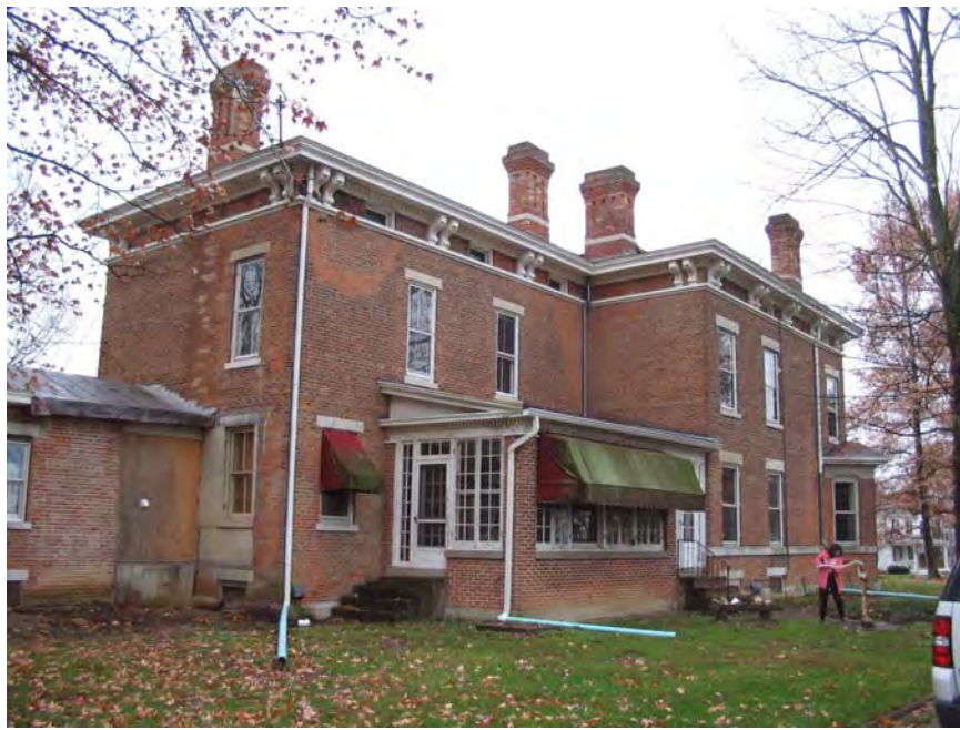
Photo 3. West and north elevations, looking southeast
