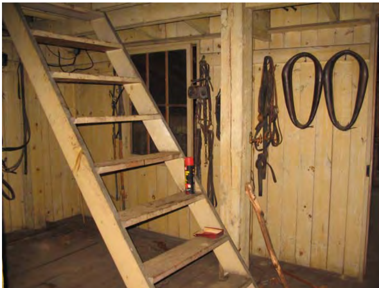
Photo 11. Attic Tack Room, looking south
