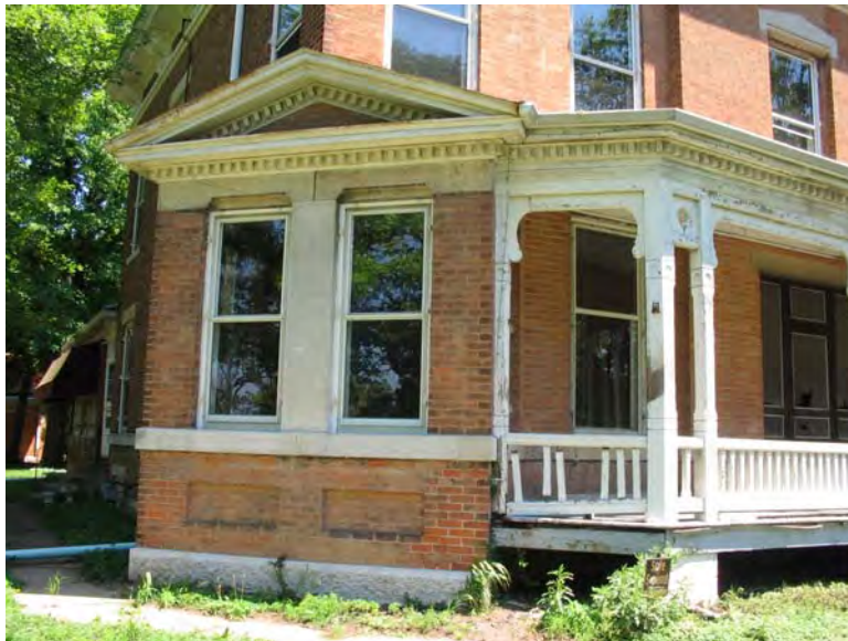
Photo 2. Southwest corner bay
